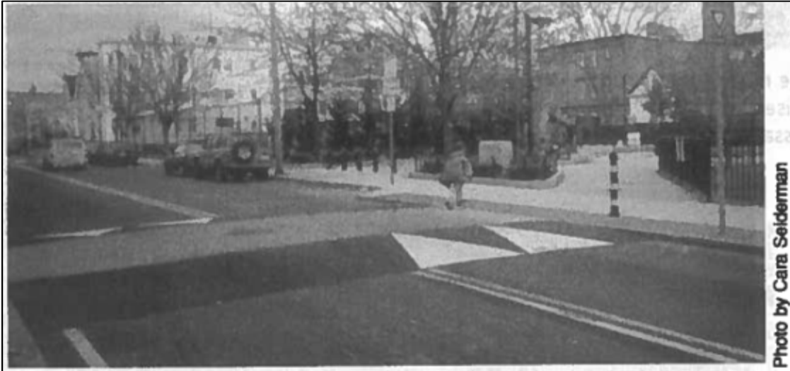
Raised crosswalk (Source: FHWA Pedestrian Facilities Users Guide).
