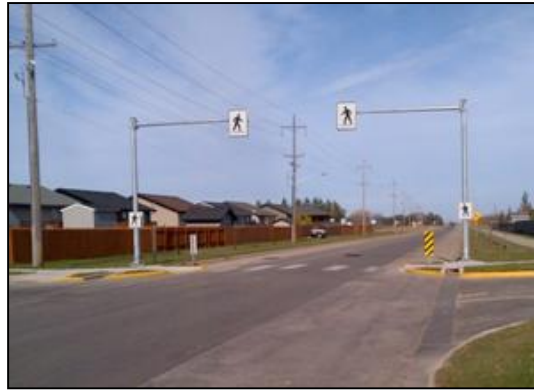
Overhead-Mounted Signed Crosswalk
