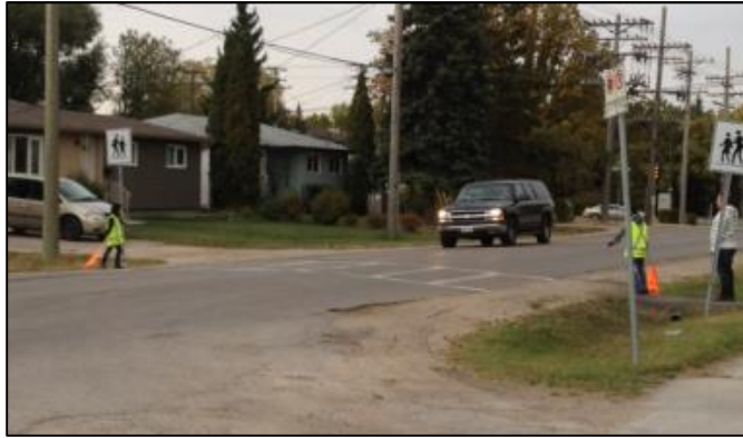
This signed crosswalk includes the RA-3 signage.
